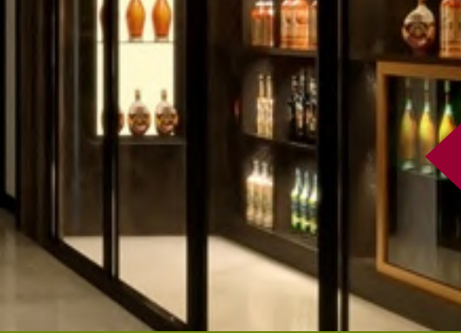
WINE ROOM WITH AIR CONDITIONING
